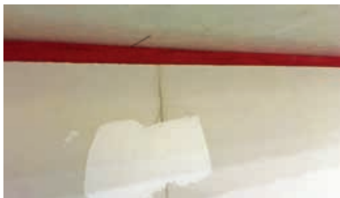
CEMCO HOTROD Compressible Firestopping is fully cured upon installations and seals off uneven concrete.
