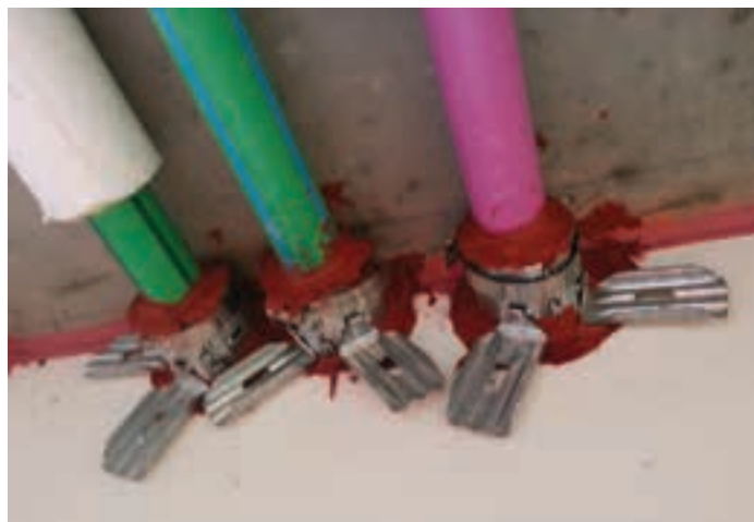
Special Inspectors will be able to assist and detect the differences between proper and improper firestop installation.
